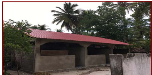
New Roof and Addition
